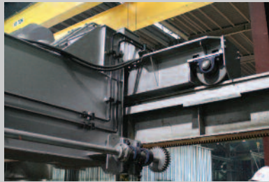
View of the Extractor's end truck during alignment.
