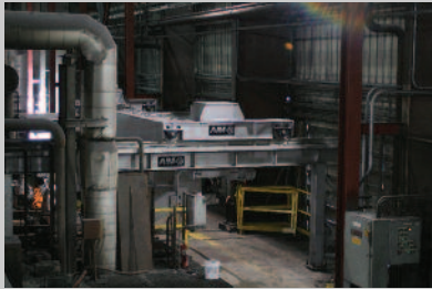
Extractor being installed.
